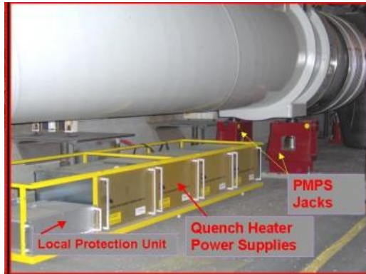
QHPS and LPU installed in LHC Quench Heater Power Supplies Local Protection Units
